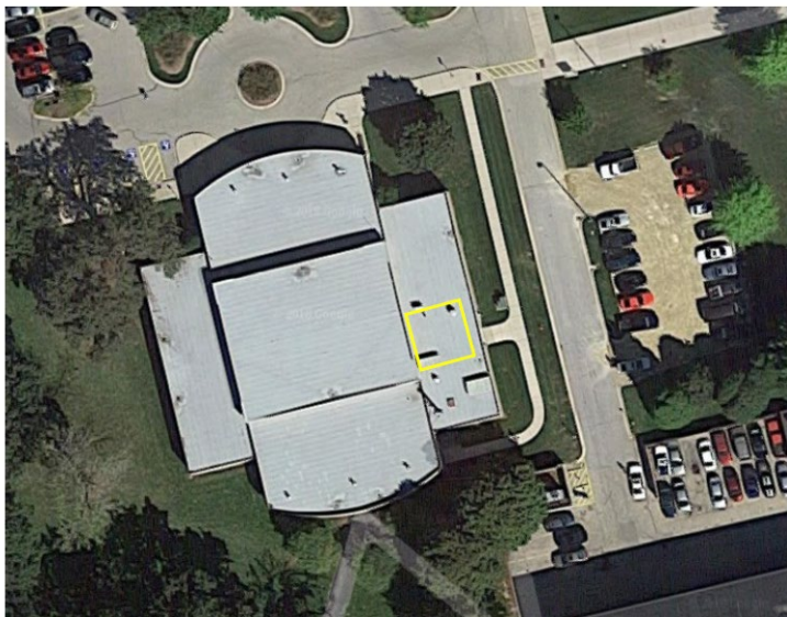
Henning Computer Center Building
