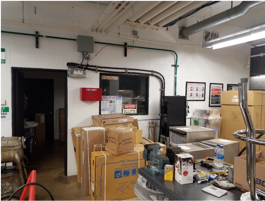
Figure 4-Area outside Room 109 entrance facing west
