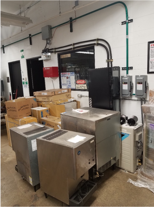
Figure 5-Area outside Room 109 entrance facing west #2
