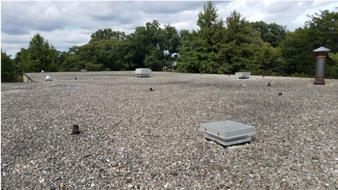
Von Ohlen Hall Roof - Facing North from BDE Roof
