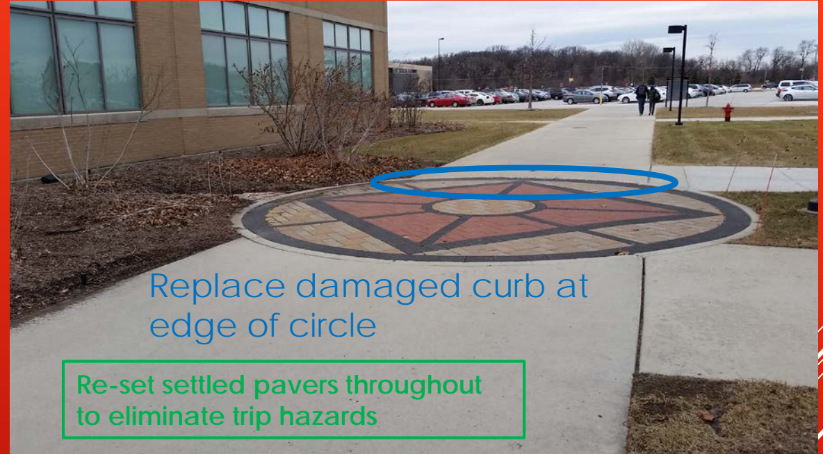
Decorative paver circle East of SCI (Near ERK)
