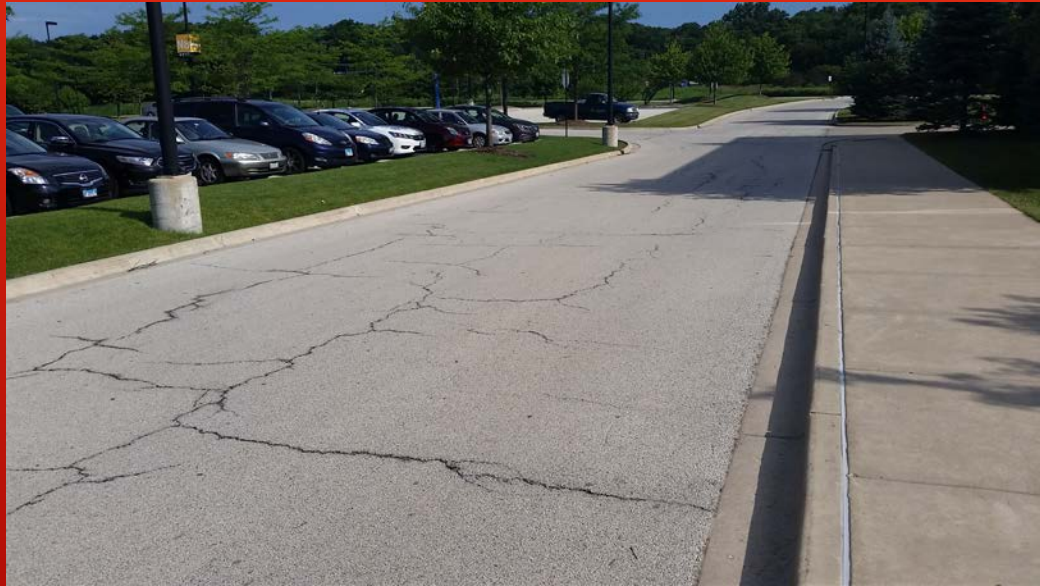
Lot N8, adjacent drives, and AKL lot – crack-filling, seal-coating & re-stripping
