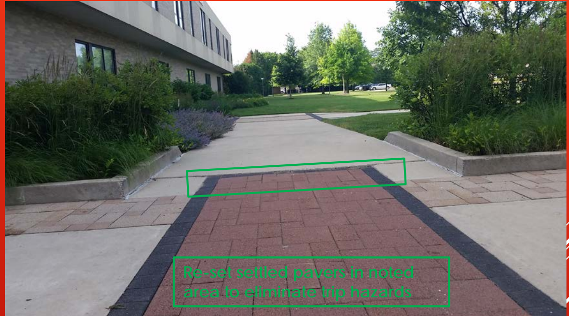
Decorative inlaid pavers West of APC building
