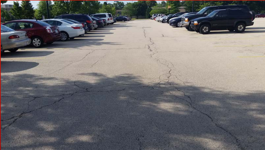
Lot N8, adjacent drives, and AKL lot – crack-filling, seal-coating & re-stripping
